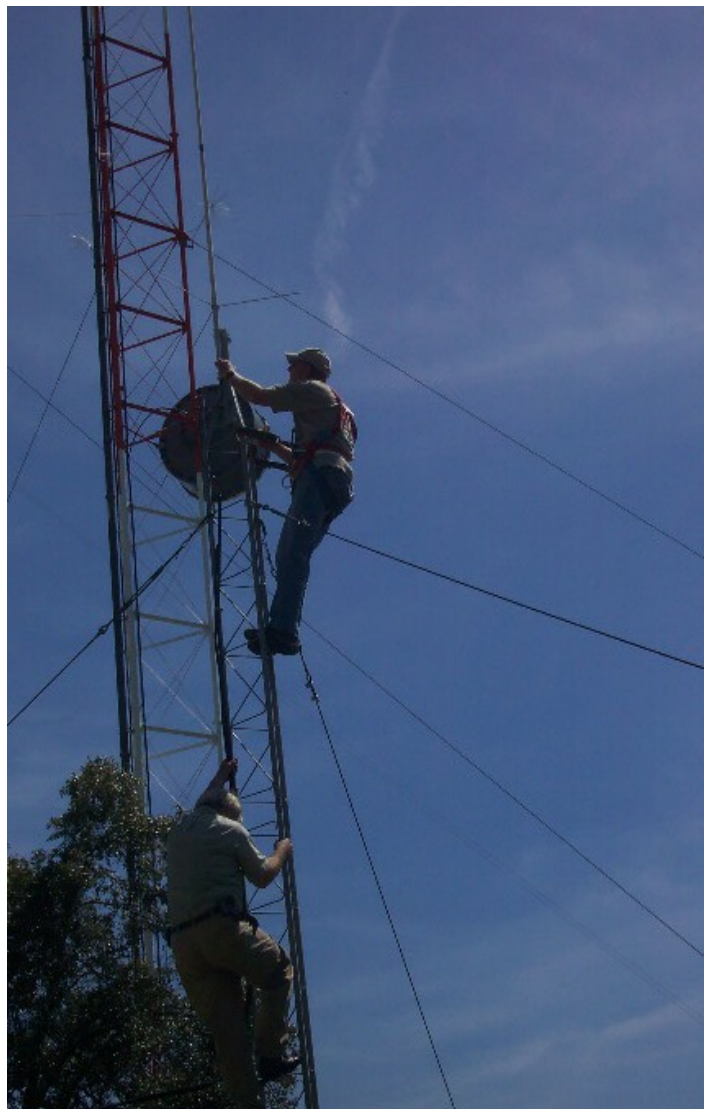
Paul W6VPS and Ken WA6OIB atop the tower removing the antennas from the old repeater site.
